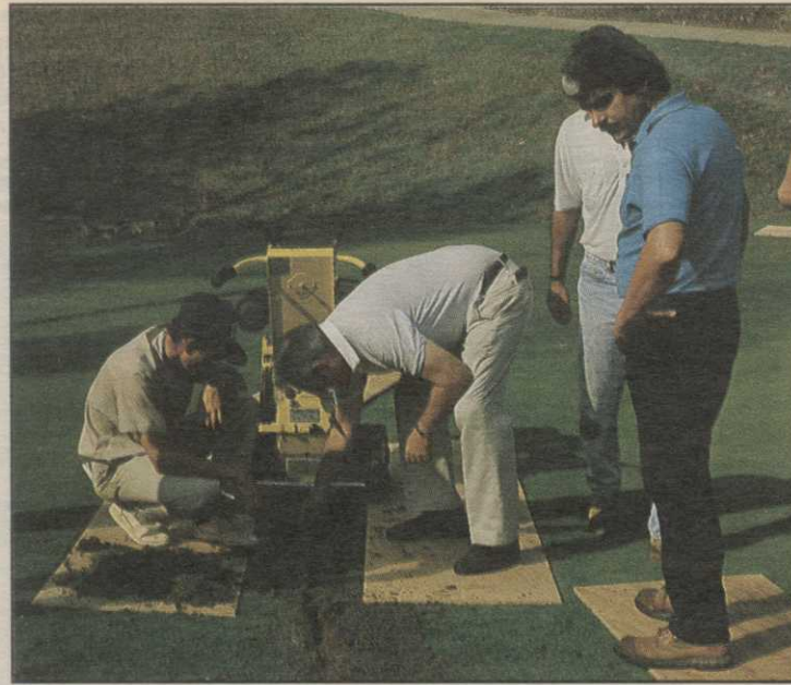
Paul Latshaw, right, oversees Greens Encroachment installation.
