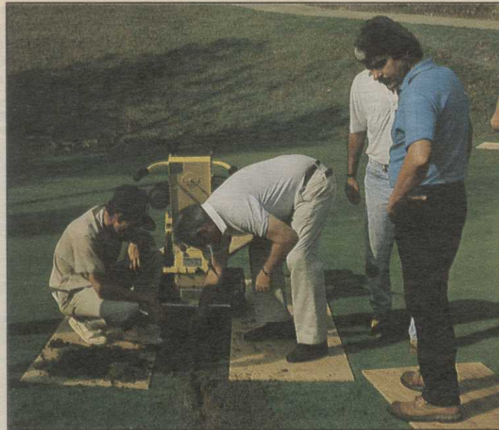
Paul Latshaw, right, oversees Greens Encroachment installation.
