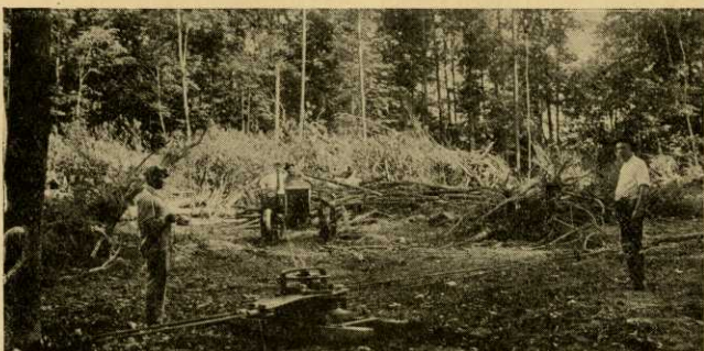
Work in Progress—New Century Golf Club, White Plains, N.Y.
