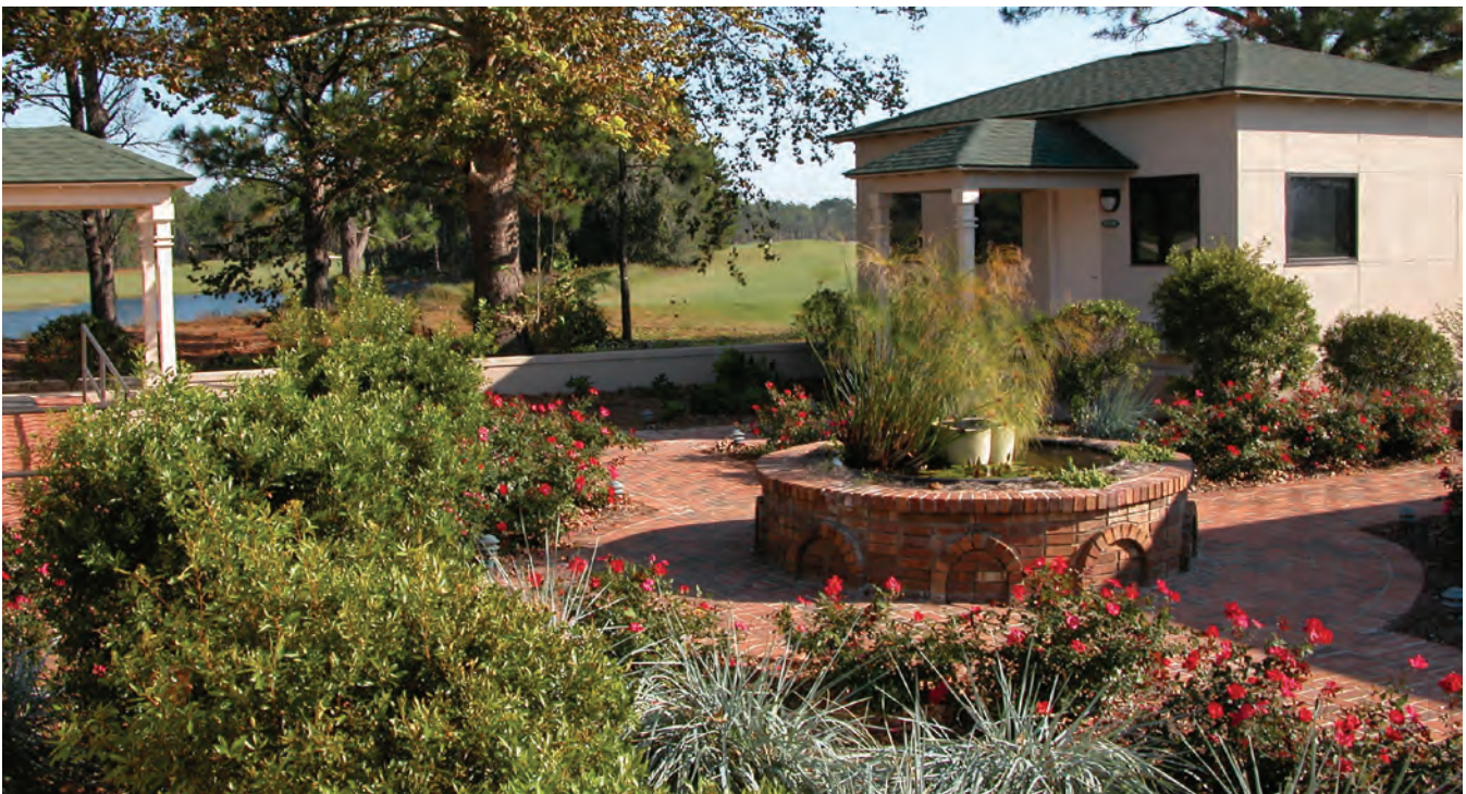
These golf villas were built on the foundation slabs of Camp Gordon Johnson's 600-foot radio tower used during World War II. Photo by Joel Jackson.
