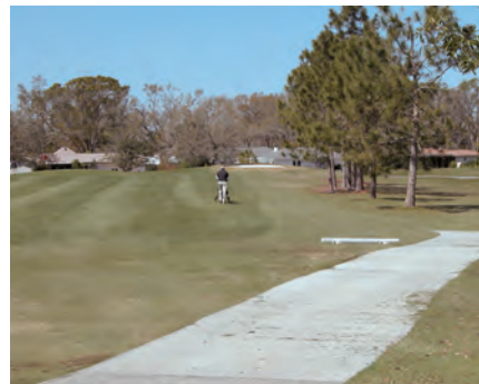
New 7-foot wide concrete paths replace and re-route the old asphalt paths. The crew often led by the owner Ed McMillin pours the new path in 110-foot long sections, which equals one truck load of concrete. Photo by Joel Jackson.
