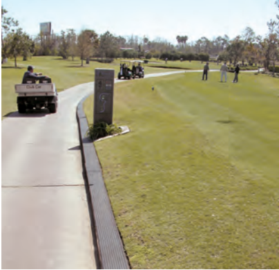
Railroad-tie curbing is installed along the new paths at the tee boxes. Non-skid rubber mat runners are installed to prevent golfer slips and falls. Photo by Joel Jackson.
