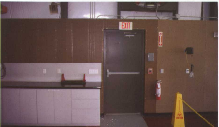
Photo 3. Pegboard wall covering in the shop helps deaden sound and keep items neatly organized and stored.
