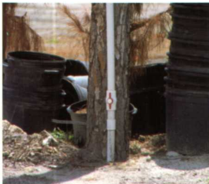
A simple, inexpensive quarter-turn ball valve controls water flow to each sprinkler. Total cost of temporary irrigation system was less than $100 to protect huge investment in plant material. Photo by Darren Davis.
