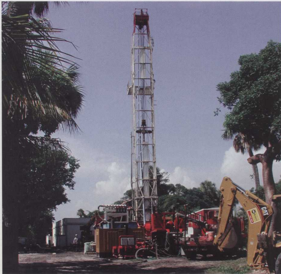
To comply with restrictions on withdrawing brackish water from the surficial aquifer during drought conditions, The Everglades Club installed a well into the deeper saline Floridan aquifer to provide water for its reverse osmosis plant to irrigate the golf course.
