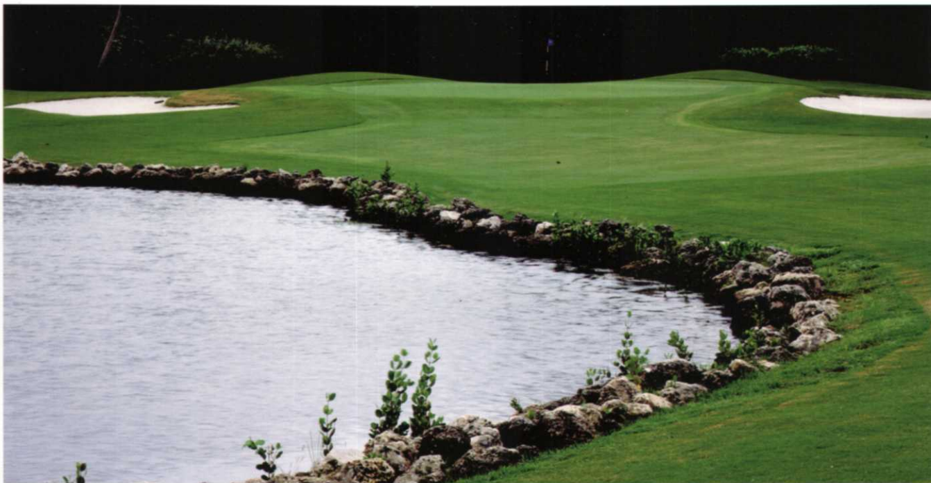
Superintendent Lee VanValkenburg had to outfox land crabs with geotextiel fabric layers and ballast stone to keep them from undermining the rip-rap lining the lake on Harbor No. 6, a 162-yard par 3. Photo by Daniel Zelazek.
