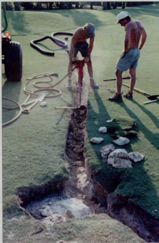
Limestone bedrock makes drainage installation a necessary but tough job.
