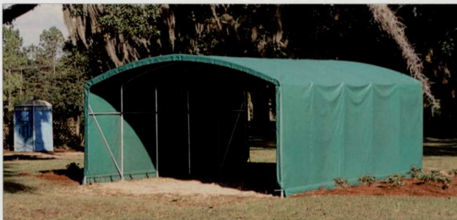
This “clear span” designed structure of galvanized steel and reinforced vinyl has proven to be an inexpensive and efficient solution to Seminole CC’s rain shelter problems. Photo by Darren Davis.
