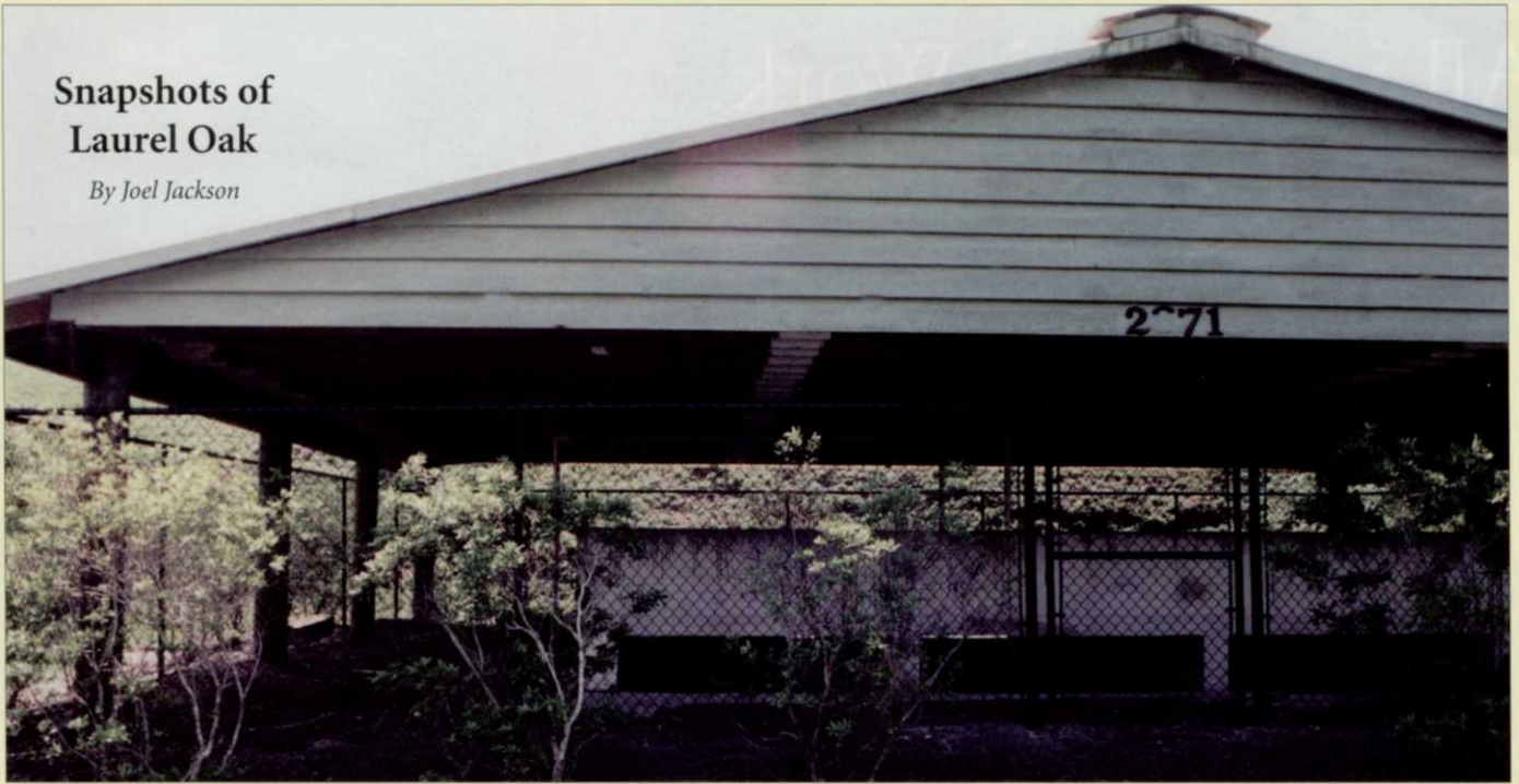
For nearly a decade this covered concrete vault system has been successfully filtering and degrading equipment washdown water and pest control rinsate.
