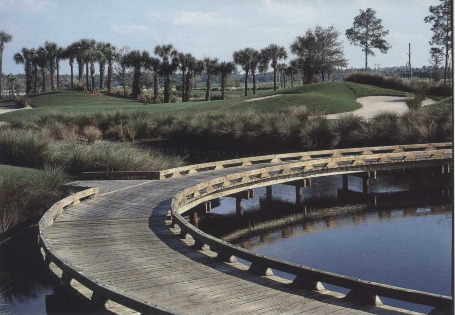
Wetland bridge ties tee and green together on hole #3. Photo by Daniel Zelazek.
