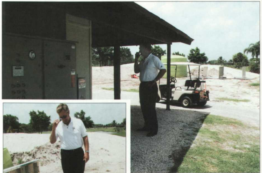
Control panels for the new Flowtronex VFD installed on the South Course are located next to an existing rest room building (above). The new pumps are housed in an underground vault in the background.
