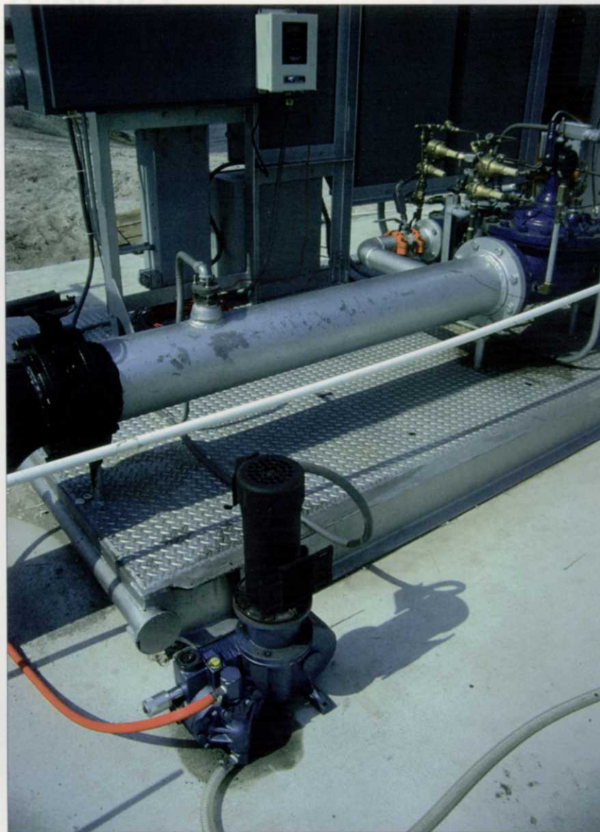
The liquid fertilizer delivery rate of the pump in the foreground is regulated by the controller in the background to provide a preset ratio of fertilizer to irrigation water regardless of the amount of water being applied. Photo by John Cisar.
