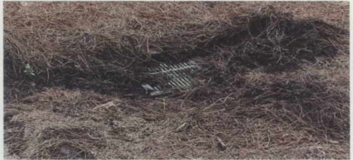
A drain basin in a depression in a pine straw area will get clogged by the moving pine straw. Photo by Joel Jackson.
