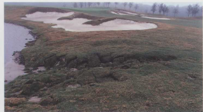
Mother nature's blowout. A phenomenon common during construction and renovation projects. It never rains hard until you lay new sod down on a slope! Photo by Joel Jackson.
