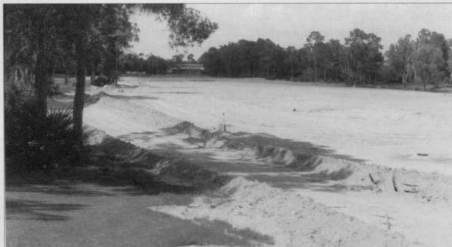
Going up — When completed, rebuilding project at The Forest will have used 42,000 cubic yards of fill to raise the level of 10 of the Bobcat course fairways, some by as much as 2 feet as shown here on No. 2. Photo by Bill Kilpatrick.
