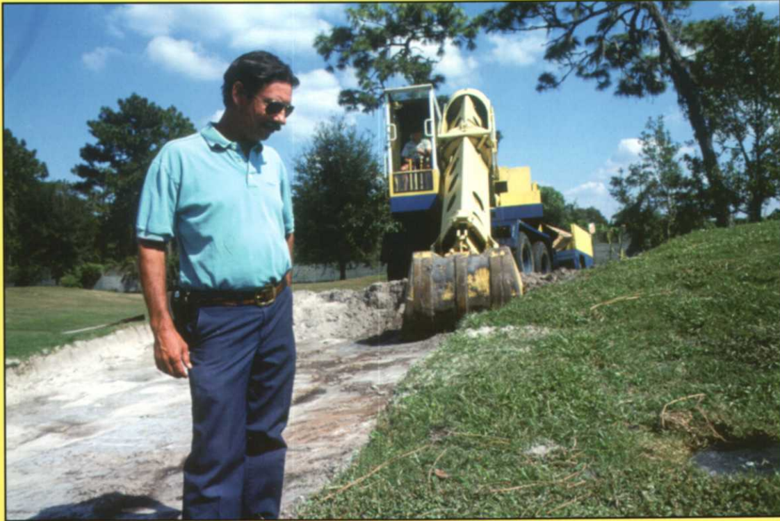
Superintendent Al Schram oversees a bunker excavation project.
