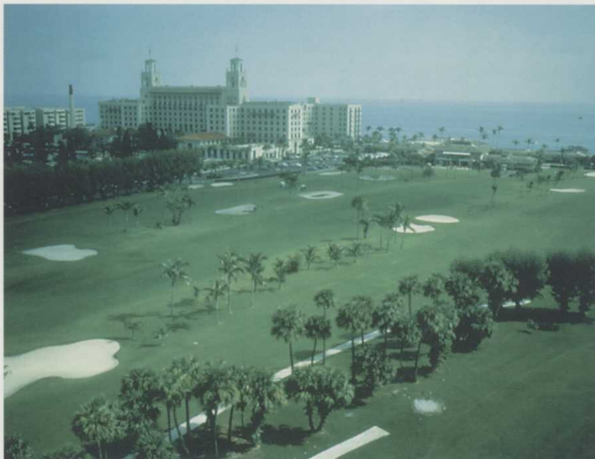
The Breakers Hotel and Golf Course was the site of the week-long conference.
