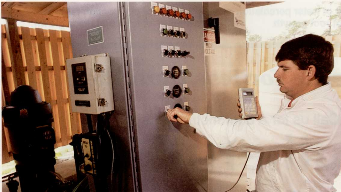
When Gator Creek Superintendent Mark Todd checks his VFD pump system, he reads the digital screen on his operator interface device (OID) and easily scrolls through complete diagnostic and historical information stored in the system.
