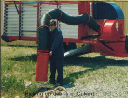
Picking up debris in Culvert
