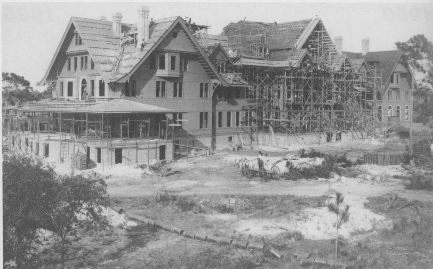
Construction of Biltmore Hotel in 1895-1896.
