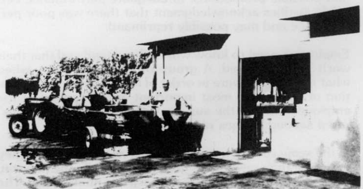
Boca Greens chemical room is designed with easy entry, concave floor with drain, sink, and outside hose bib. ■
