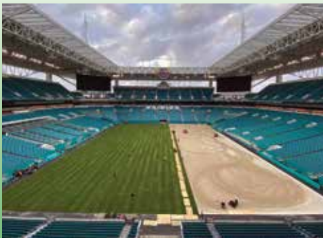
Construction of Super Bowl LIV Field, 2020
