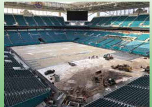
Hard Rock Stadium SubAir Drainage Installation
