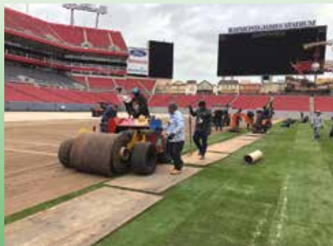
Construction of Super Bowl LV Field, 2021
