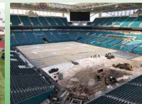
Hard Rock Stadium SubAir Drainage Installation
