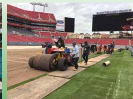
Construction of Super Bowl LV Field, 2021
