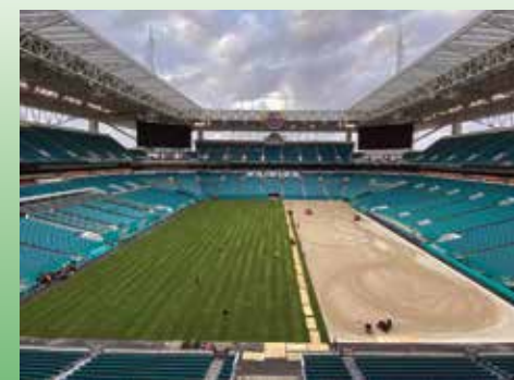
Construction of Super Bowl LIV Field, 2020
