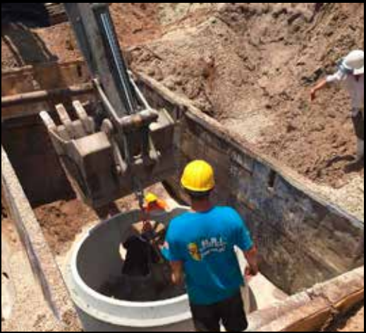
New Wet Well Construction
