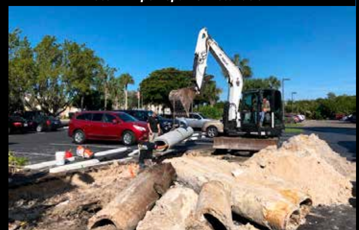
Storm Pipe Repair & Installation
