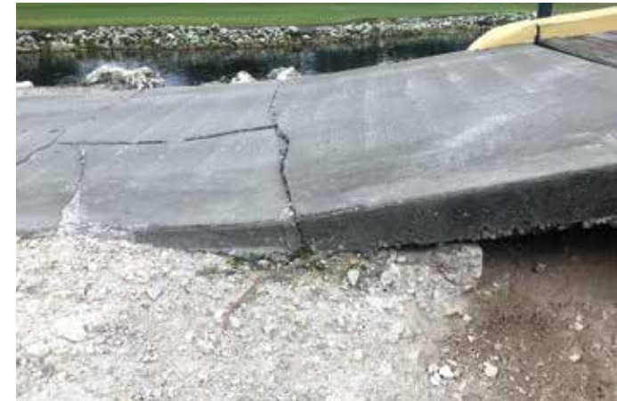
Burrowing iguanas can undermine bridges leading to extensive damage.
