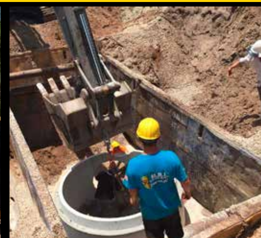
New Wet Well Construction
