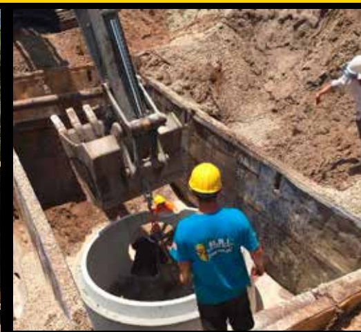
New Wet Well Construction
