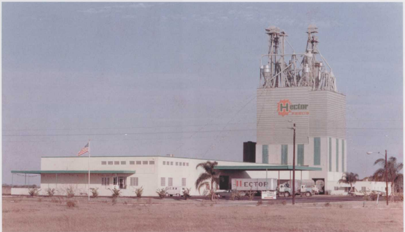
Hector Fertilizer Plant. The company sold its farm supply and fertilizer business interests in 1969.
