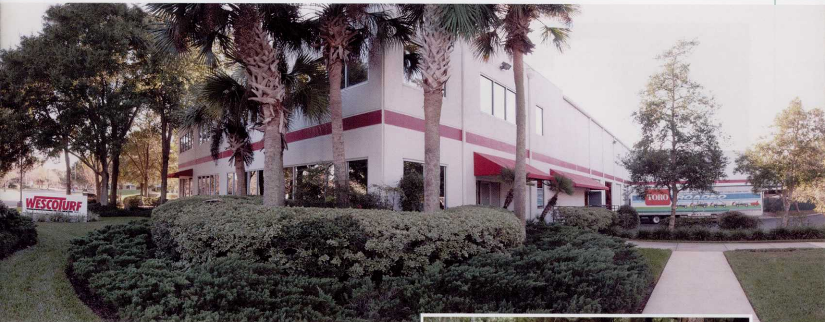
The Wesco Turf, Inc. regional headquarters: The picture on the left is the Sarasota office; the one above is the Lake Mary office. Submitted by Billy Gamble
