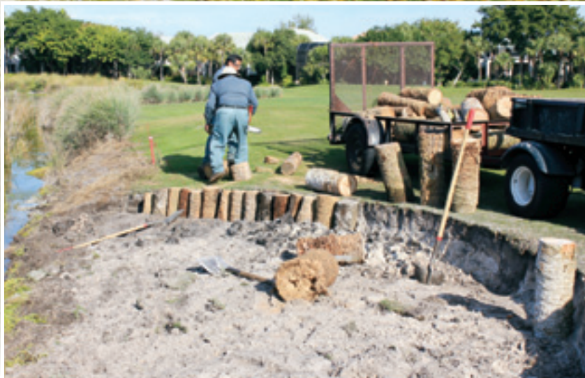
Above: Sanctuary crewmembers building a protective gator beach area. At top left: Gator sunning on a beach created on The Sanctuary Club. Photos by Kyle Sweet.
