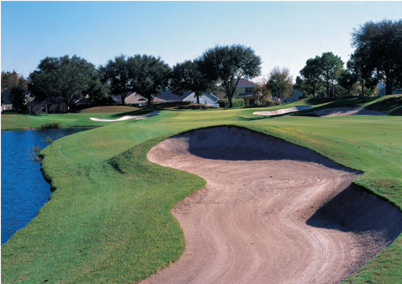
This steep-faced bunker on No. 14 is among the fairway bunkers slated for reconstruction to improve drainage and prevent washouts. Photo by Daniel Zelazek.
