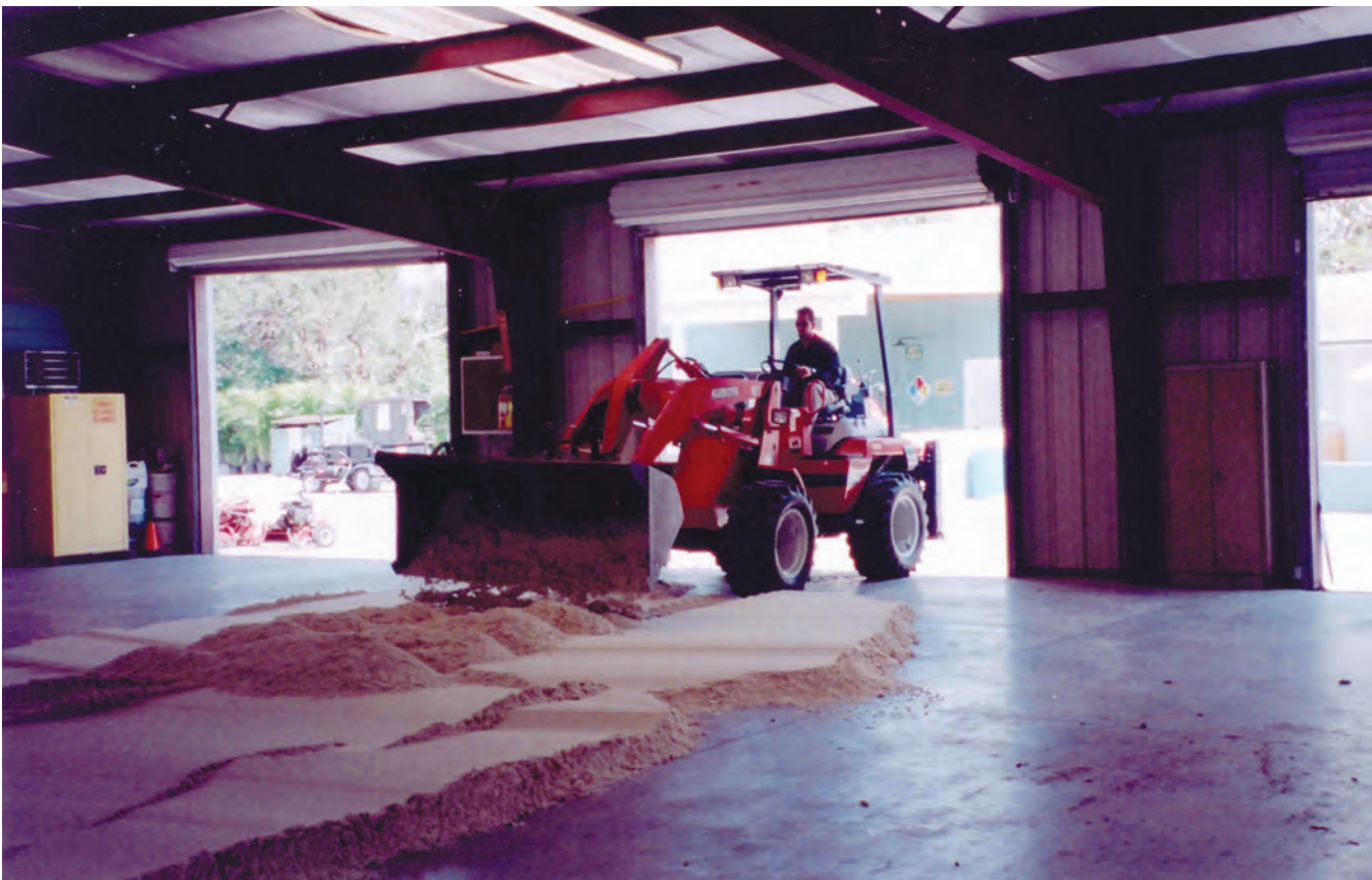
How to build a beach. Start with 20 tons of sand and an empty maintenance building.
