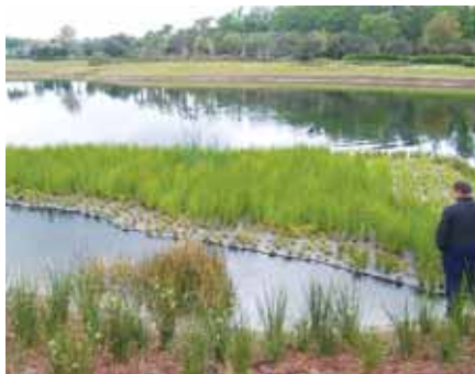
This particular mat at Twin Eagles had broken away from its anchor and Sean graciously left it where it was so that Todd and I could get a first-hand look at how it was put together. Photo by Shelly Foy.
