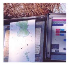
Simple laminated hole drawings mounted at each satellite makes learning irrigation zones and problem areas easier. The black numbers are the controller station numbers and the red numbers indicate heads with yardage plates on them. Photo by Darren Davis. camera. I had each crew member stand against a blank wall and I took individual head-and-shoulder photos. I downloaded the files to my computer and formatted them to print on Kodak photo paper, with each photo measuring 2 by 2 inches.
