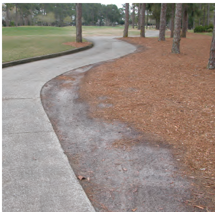
Sweeping curves in a cart path are very aesthetic looking but drivers cut them short and create worn turf and potholes. Photo by Joel Jackson.
