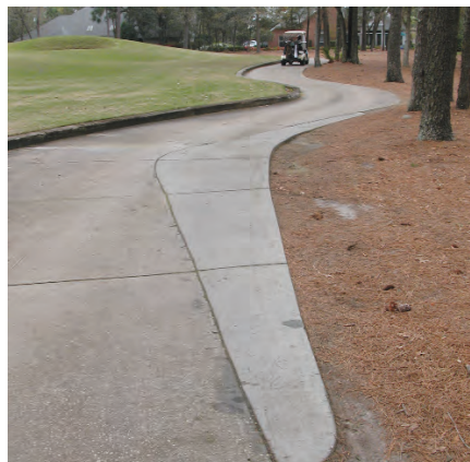
To avoid future potholes many courses add pavement to the curves. Photo by Joel Jackson.
