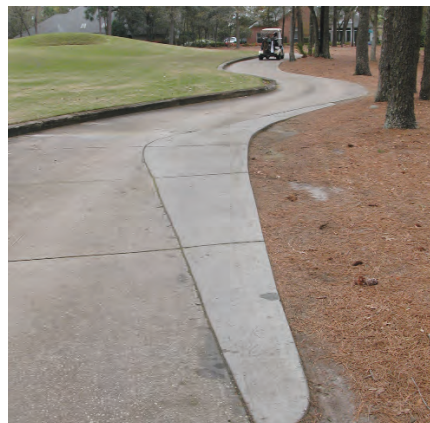
To avoid future potholes many courses add pavement to the curves. Photo by Joel Jackson.
