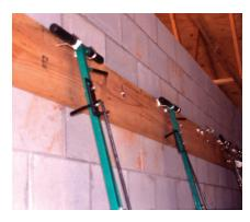
Hanging around: Need more room in your facility, but have fertilizer spreaders taking up valuable floor space? At Reynolds Plantation in Georgia a 2 by 8 plank was anchored to the concrete wall and steel hooks were screwed into the full depth of the wood, allowing a quick, easy and inexpensive solution
