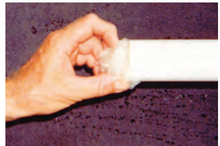
Insert water-soluble material into pipe to block flow. The material will dissolve completely and not plug up sprinklers.
