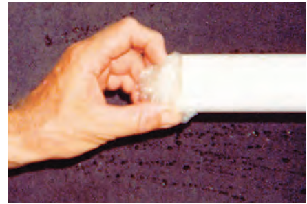
Insert water-soluble material into pipe to block flow. The material will dissolve completely and not plug up sprinklers.
