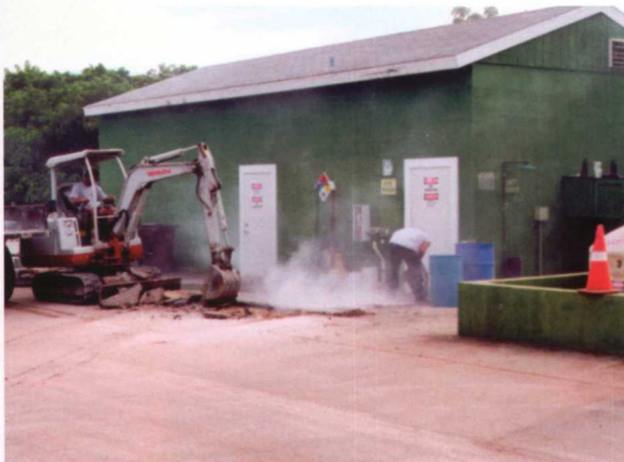
Demolition of the old slab outside the chemical room. Note containment around the fertigation tanks to the right.
