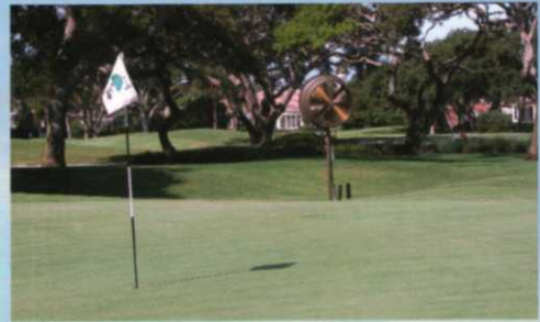
An oscillating fan was installed on No. 6 South to combat shade induced dampness on the green.
