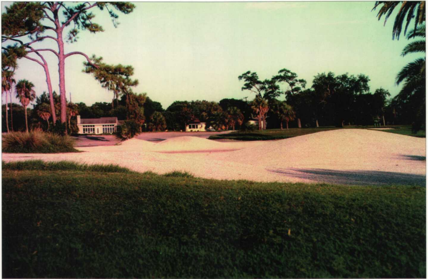
This formerly sandy soil waste bunker between holes #3 and #4 is being converted to a crushed oyster shell material. This crushed material, similar to coquina gravel, provides a better playing surface to hit from and requires less maintenance for grooming. Photo by Joel Jackson.
