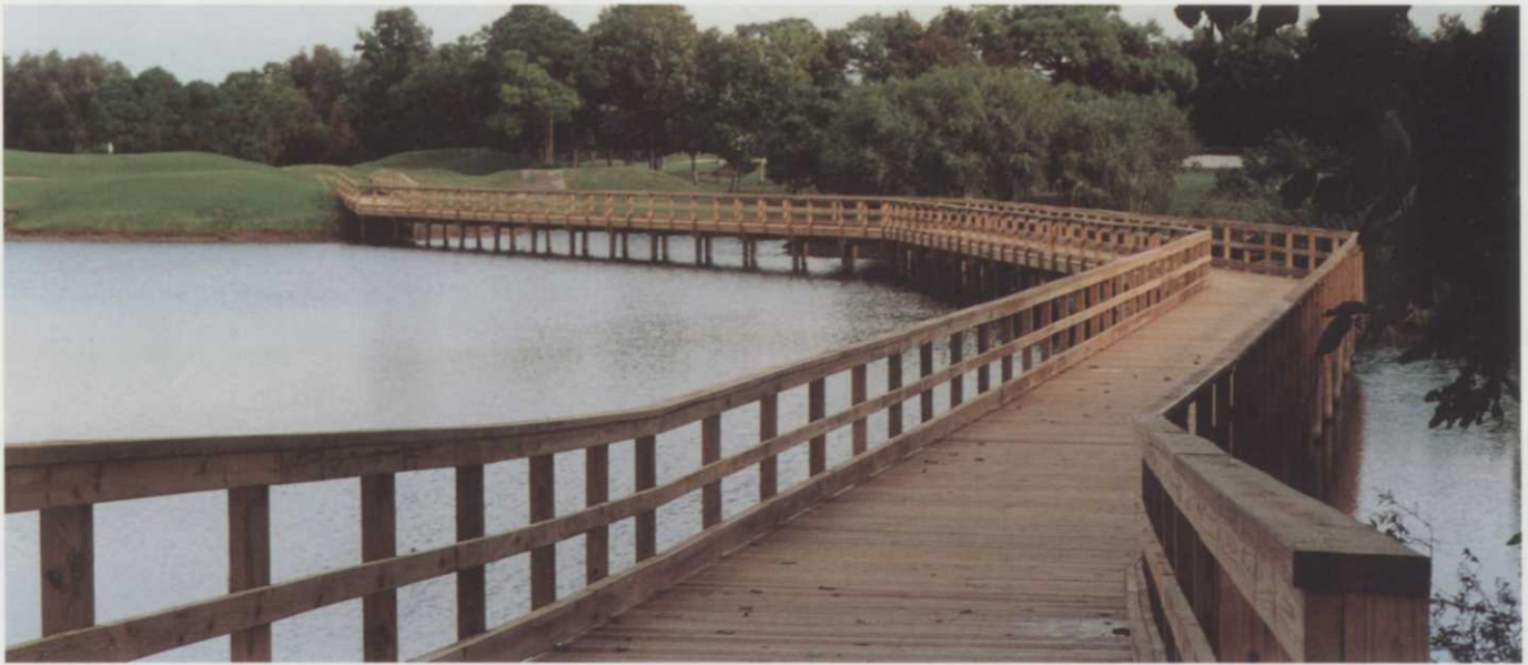
This 405-foot-long bridge at Admiral's Cove may be one of the world's longest wooden golf cart bridges. Photo by Bill Brousseau.
