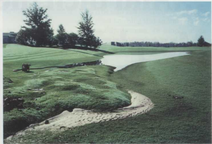
An irrigation blowout. Usually an overnight occurrence that greets you in the morning with a flood, a mound or a hole and lost irrigation coverage to deal with. Photo by Joel Jackson.
