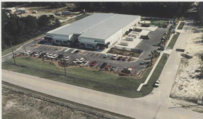
The Kilpatrick Company in Boynton Beach has a new facility which includes the one-hole Turtle Ridge Golf Club. The hole runs behind the building. Photo by Smith Aerial Photography.
