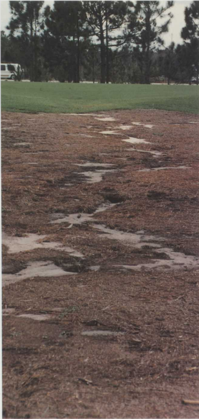
Superintendents are often called upon to correct flaws in a course design. Pine straw on a bare slope moves downhill in a heavy rain. That's not Murphy's Law. That's the Law of Gravity. Photo by Joel Jackson.
