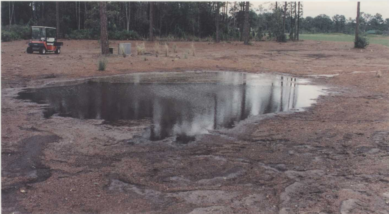
A clogged drain basin produces an unexpected water hazard. Superintendents have been known to take off their shoes and roll up their pant legs and wade in to solve the problem temporarily. Eventually the sloping pine straw areas are sodded, and work turns to more important jobs, like grooming the turf. Photo by Joel Jackson.
