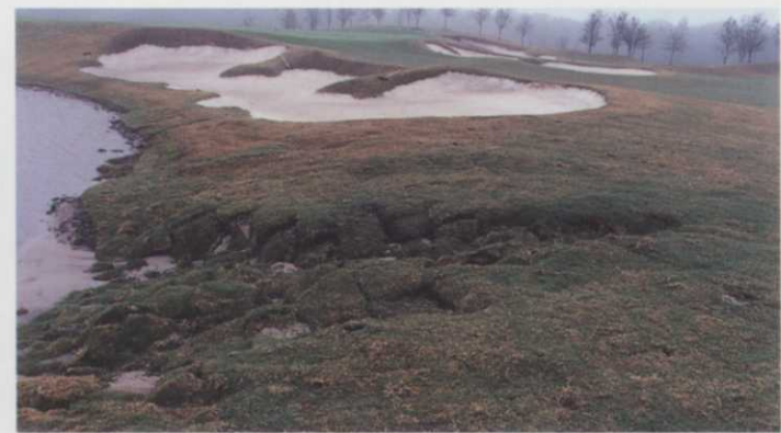
Mother nature's blowout. A phenomenon common during construction and renovation projects. It never rains hard until you lay new sod down on a slope! Photo by Joel Jackson.
