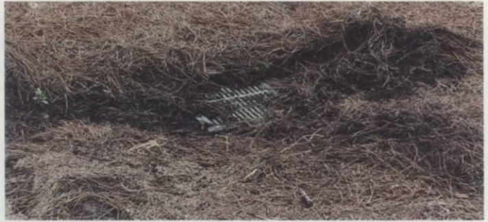
A drain basin in a depression in a pine straw area will get clogged by the moving pine straw. Photo by Joel Jackson.
