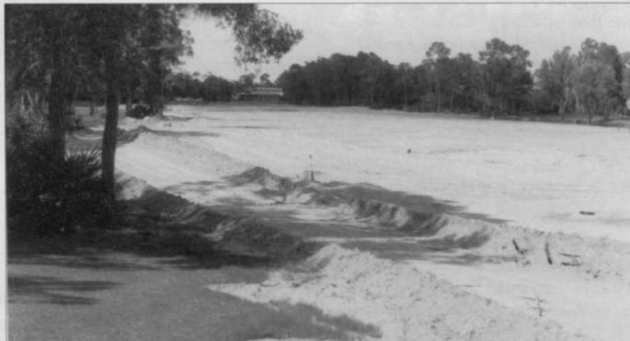
Going up — When completed, rebuilding project at The Forest will have used 42,000 cubic yards of fill to raise the level of 10 of the Bobcat course fairways, some by as much as 2 feet as shown here on No. 2. Photo by Bill Kilpatrick.
