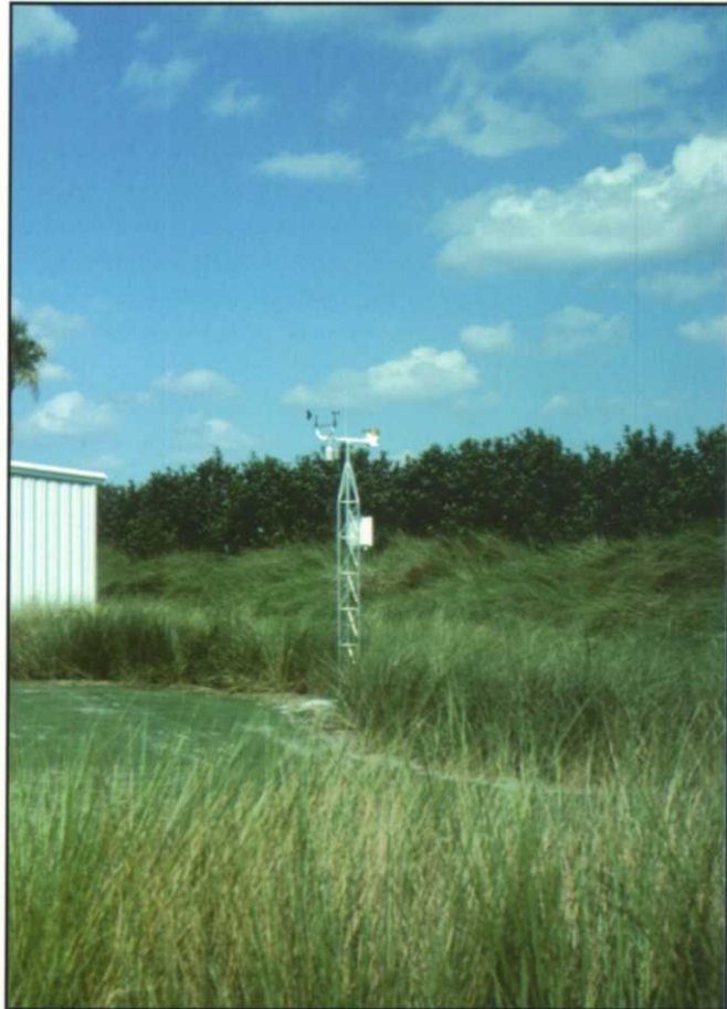
Irrigation weather station monitors conditions and adjusts run times.
