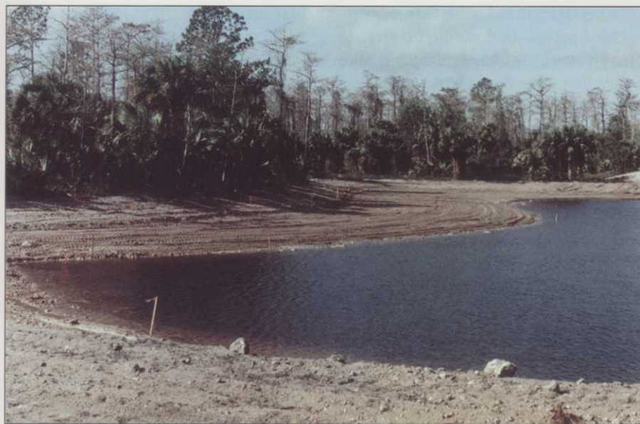
Wetland planting area during construction at Olde Florida Golf Club, Naples
