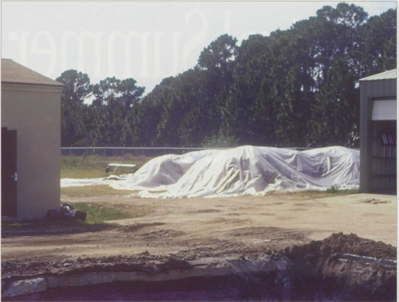
Contaminated soil must be stored on site until lab results determine the best disposal method. Extremely contaminated soil must be hauled to an approved burn center — a very expensive proposition.
